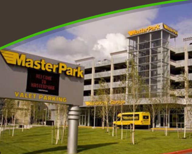
MasterPark Garage, SeaTac, WA
