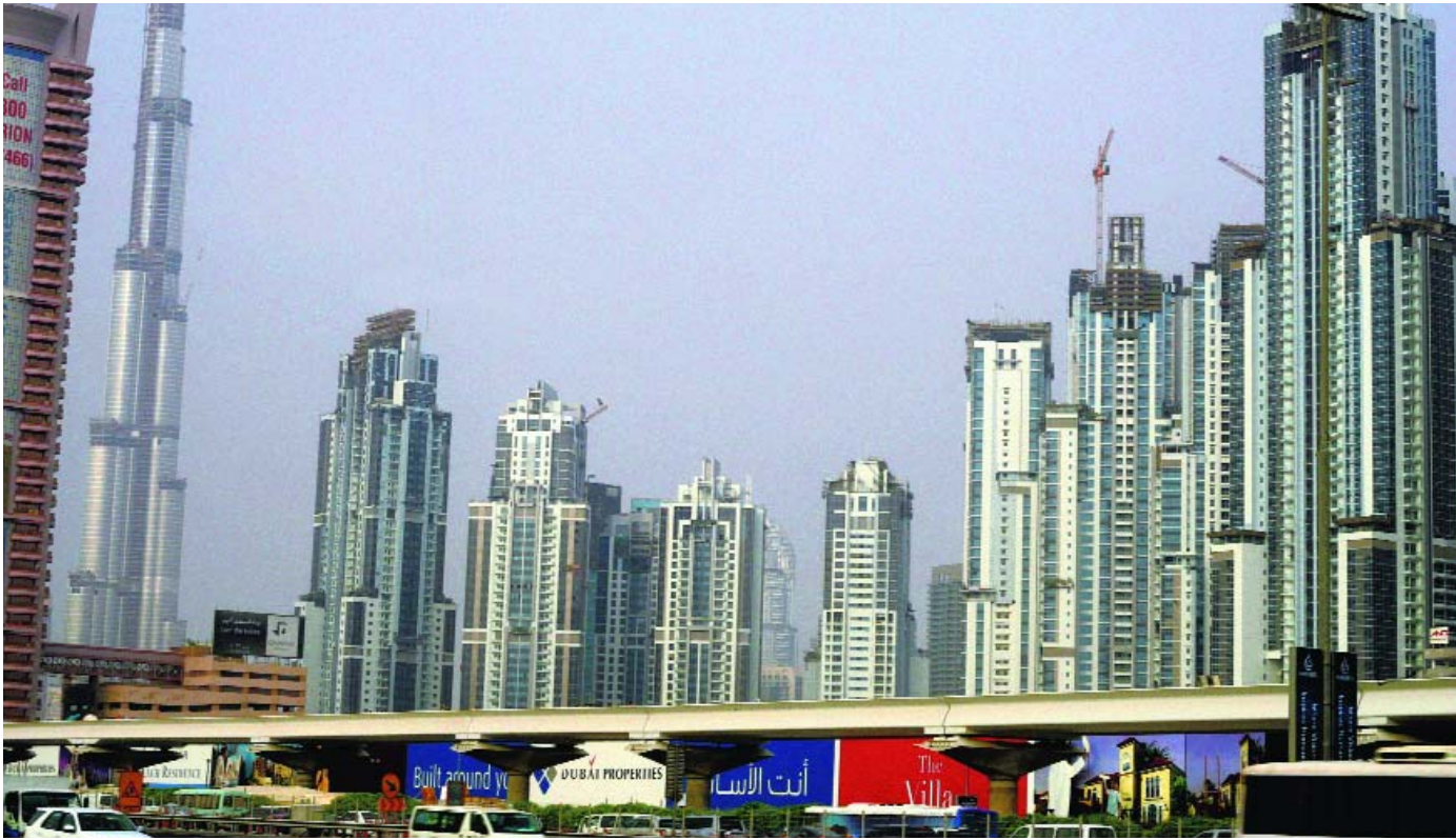
■ According to Rosenberg, Dubai has a vision of standardising green construction regulations and will soon be a green destination
